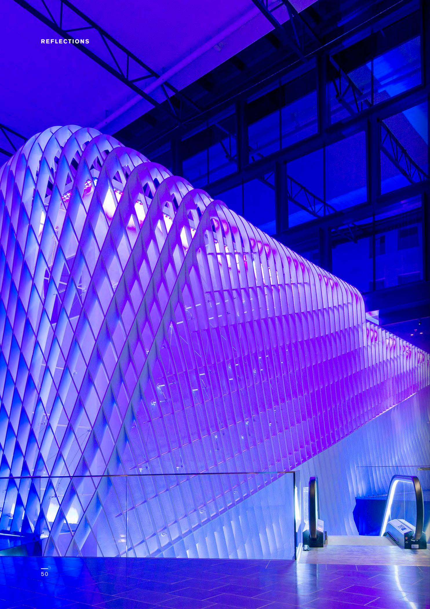
The wall cladding system for the Quality Hotel Globe foyer used computational design systems for the design of the geometry and the management of fabrication and assembly processes (left page).
