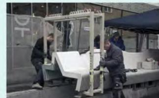
The production and assembly documentation for the Forumtorget Bench was produced directly from the computational design system developed, and a custom assembly jig was designed by the team.
