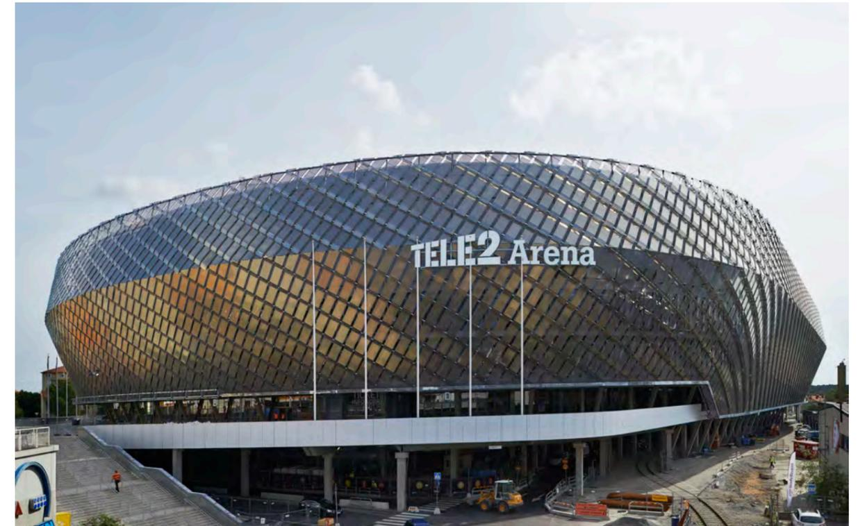
The envelope for Tele2 Arena was developed through computational design systems, providing a rational process for the design, production, and assembly (left page and above).
